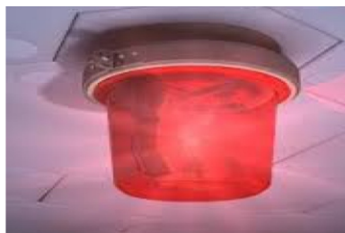
Fig. 6.1.1.4: Emergency signal lamp
